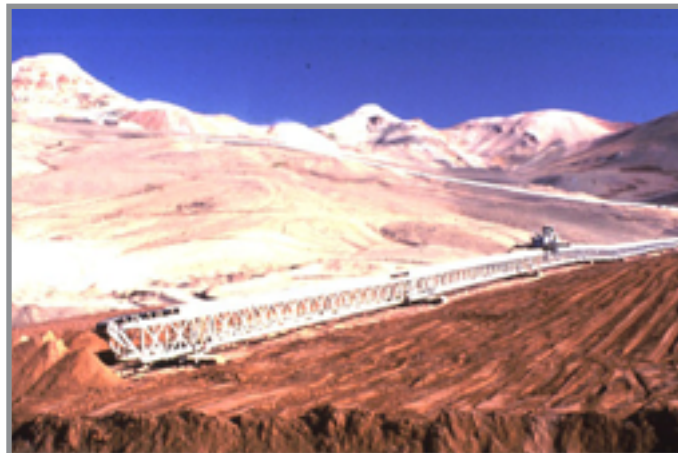
Dry tailings disposal method, La Coipa mine, Chile PHOTO: Tailings.info
